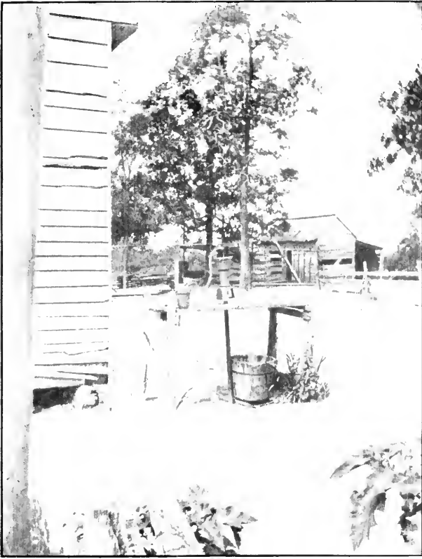
PLATE XII.—DRILLED WELL CONVENIENTLY NEAR THE HOUSE.
